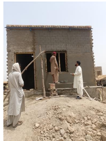
12 - Plaster work in progress
