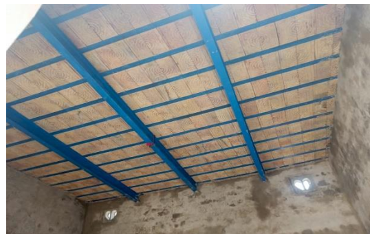
4 - View of Roof Laid used T-iron and Girder
