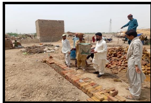
6 - Bricks curing at site
