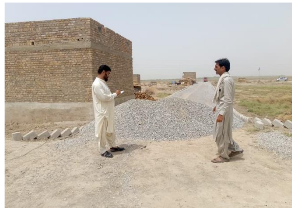
10 - View of under progress path way
