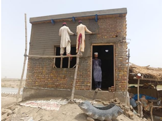
7 - Finishing/Plaster works in progress
