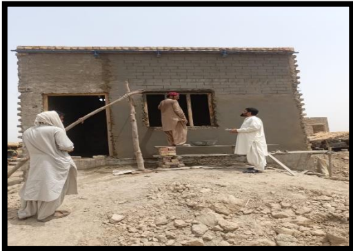
1- Finishing work in progress
