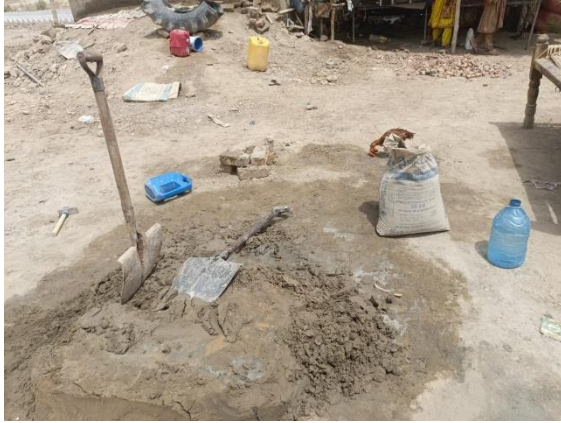
13 - View of mortar at site
