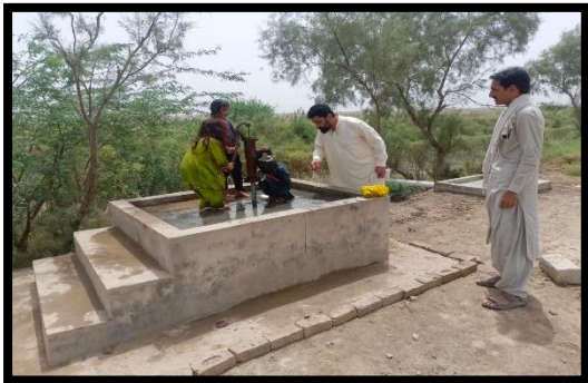
3 - View of Handpump and Washing Pad
