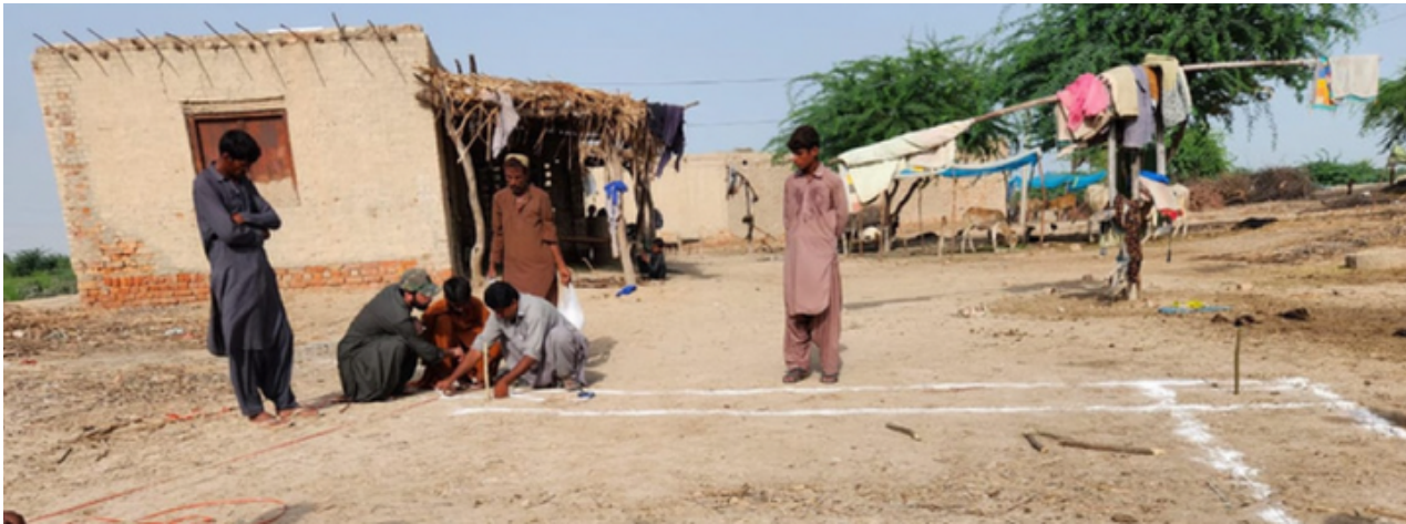
Boundary demarcation process for house construction
